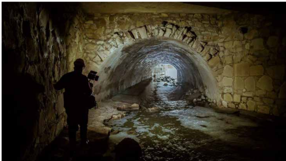
Figure 9. General view section of the stone underground culverts-arch's (Tavera, 2018)
