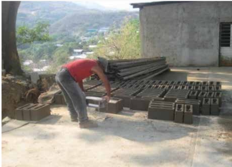
Image 12. Storage and drying. Source: Own elaboration
