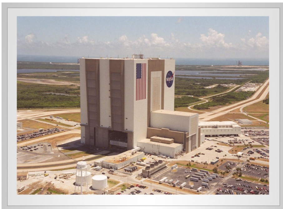
Figure 4. The Vehicle Assembly Building (VAB) was built for the Apollo program (1964). The VAB was designed to store and assemble the 110 meter tall Saturn V rocket. One of the most notable characteristics of the VAB is its 139 meter tall doors (they are the tallest doors in the world). The VAB is also used to mount the NASA Space Shuttle. The VAB is used for the mounting and assembly of the SLS and the MPCV. Photo courtesy of NASA.
