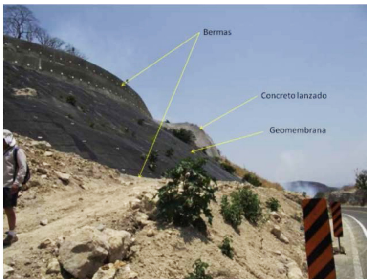
Image 4 Case 1. Ocozocoutla-Arriaga motorway (190 D) (Photo 1). Location: km 25 (16 ° 41'54.36 "N, 93 ° 32'32.56" W). (Photo 1). The zone corresponds to the contact of two units: Tritic-Jurassic shale-sandstone and lower Cretaceous limestone-shale.
