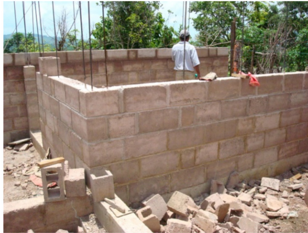
Image 9. Intermediate horizontal reinforcement
