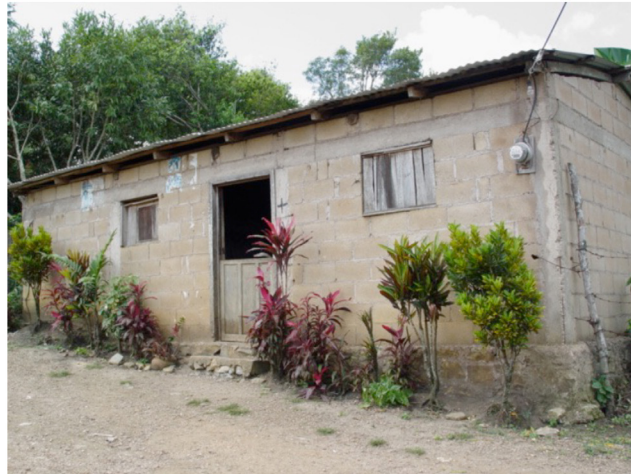
Image 3. Typical house with hollow block walls.
