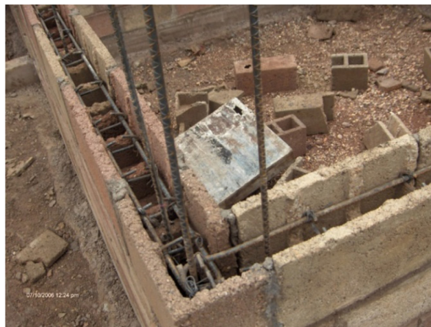
Image 9. Intermediate horizontal reinforcement
