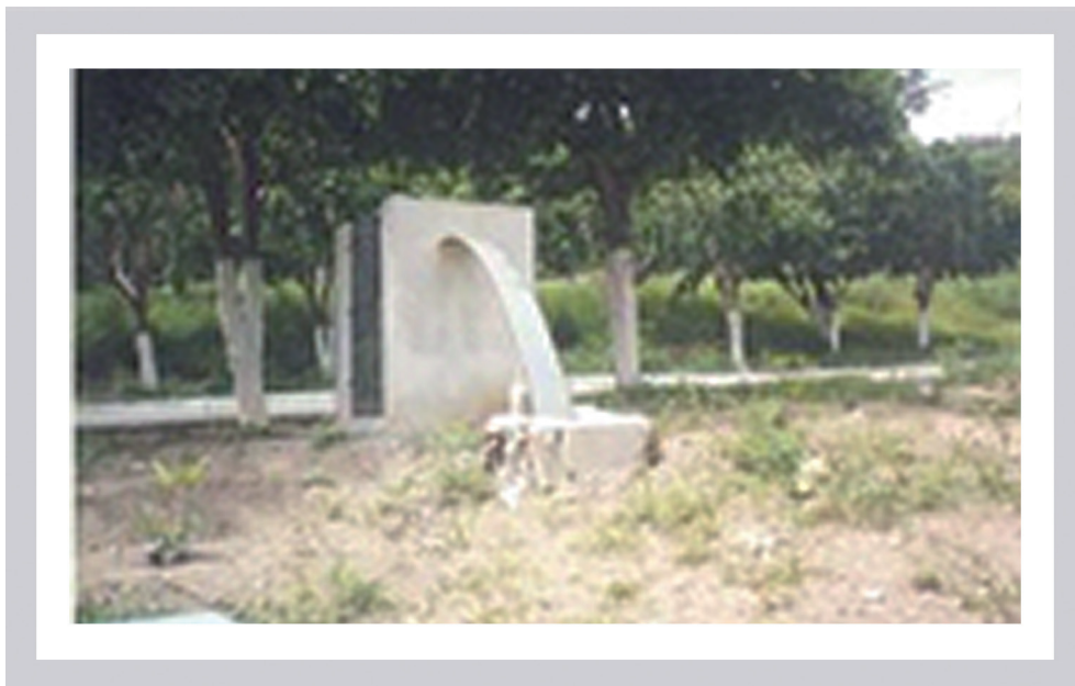
Photo 10. Laminate siphon tank
