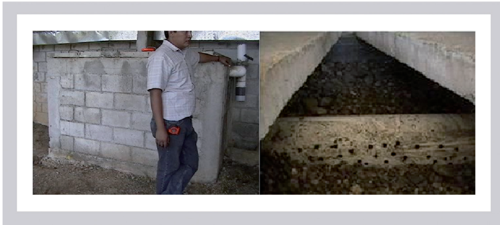
Photo 7. Sand and gravel filters in Yalentay
